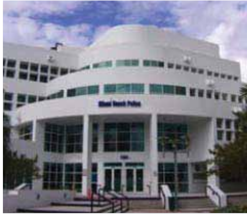
The City of Miami Beach Police Headquarters will have a geothermal plant built on-site.
